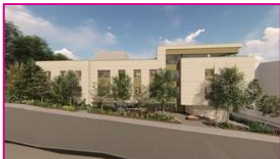
Our new Highgate East inpatient facility will open in early 2024
